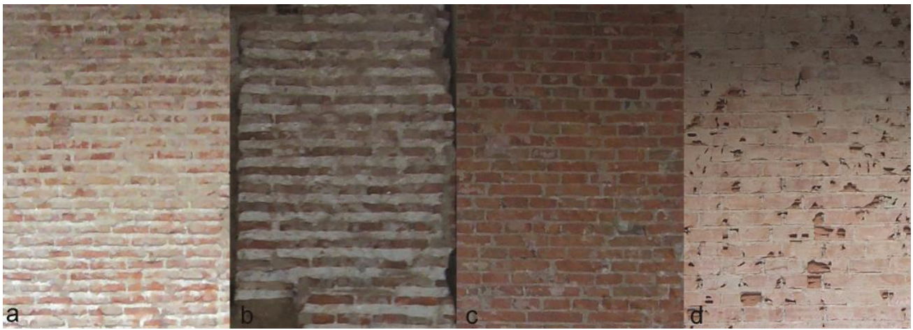
Fig. 3. Different brick morphology identified in the building: a) type i. b) type ii. c) type iii. d) type iv.
