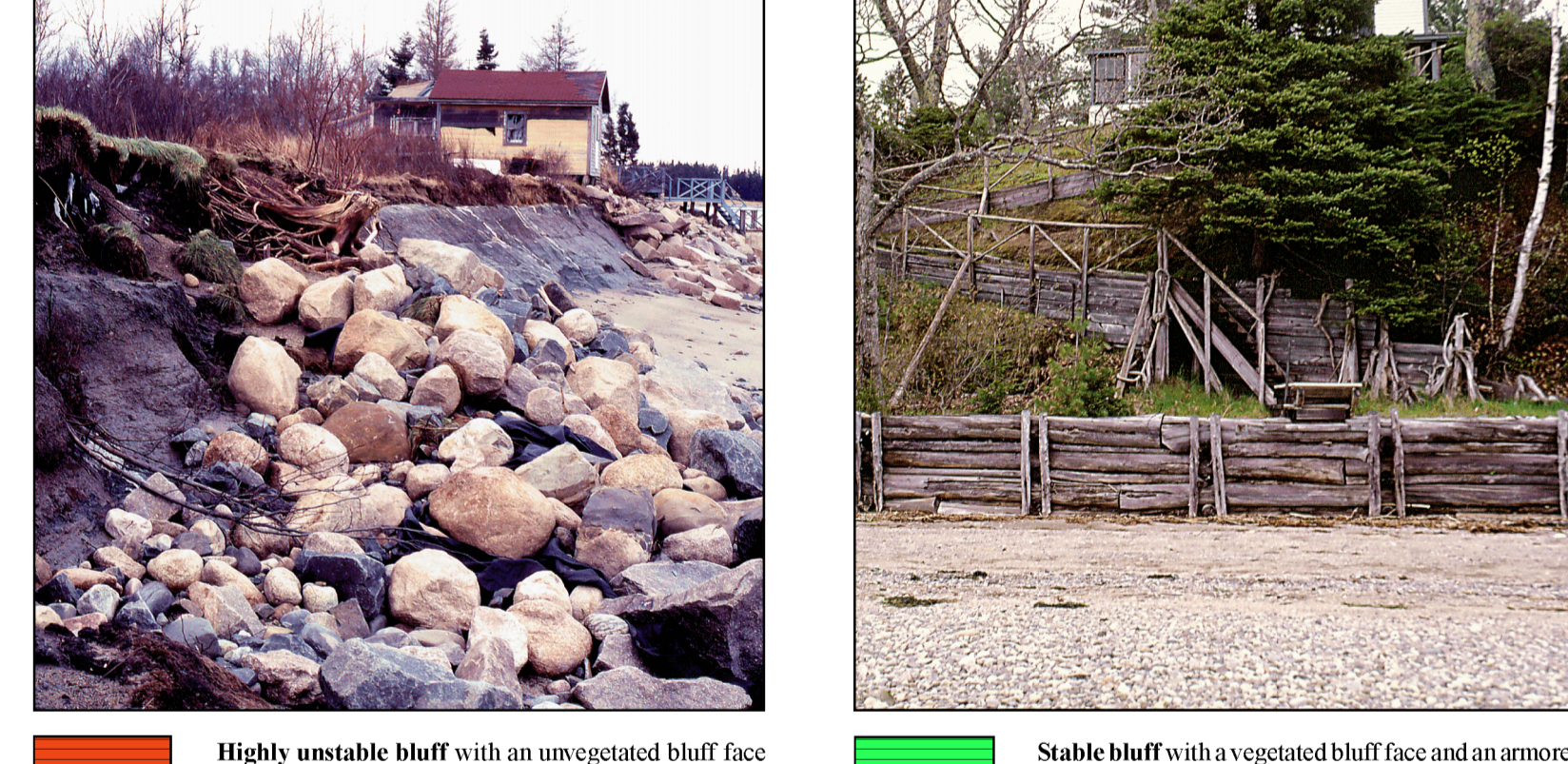
Highly unstable bluff with an unvegetated bluff face and an armored shoreline. This armored bluff is eroding despite an effort to shore it up with riprap, or loosely piled stone blocks. Maintenance at this site could improve bluff stability. Stable bluff with a vegetated bluff face and an armored shoreline. The bluff face is fully vegetated and supports a mature stand of trees with vertical trunks. The presence of a wooden bulkhead suggests that erosion has occurred in the past.
