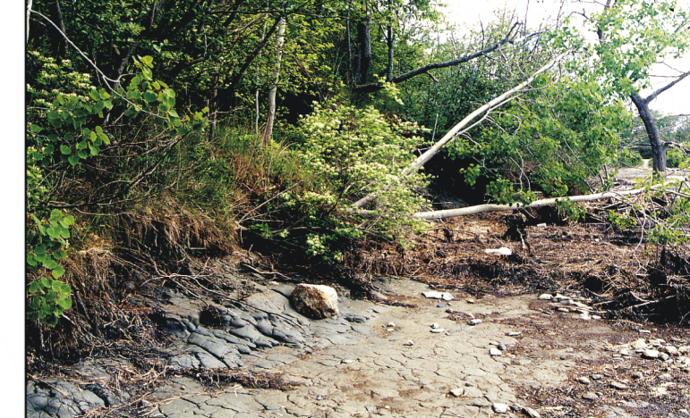
Figure 6. Wave erosion at the base of a bluff removes slope sediment and steepens the bluff. Erosion has undercut the trees in the photo above and caused them to tilt toward the ocean. This steepening reduces the stability of the bluff, and a landslide may result. Ongoing sea-level rise along the Maine coast will cause wave erosion at the base of coastal bluffs and continue to make some coastal bluffs at risk of experiencing a landslide.
