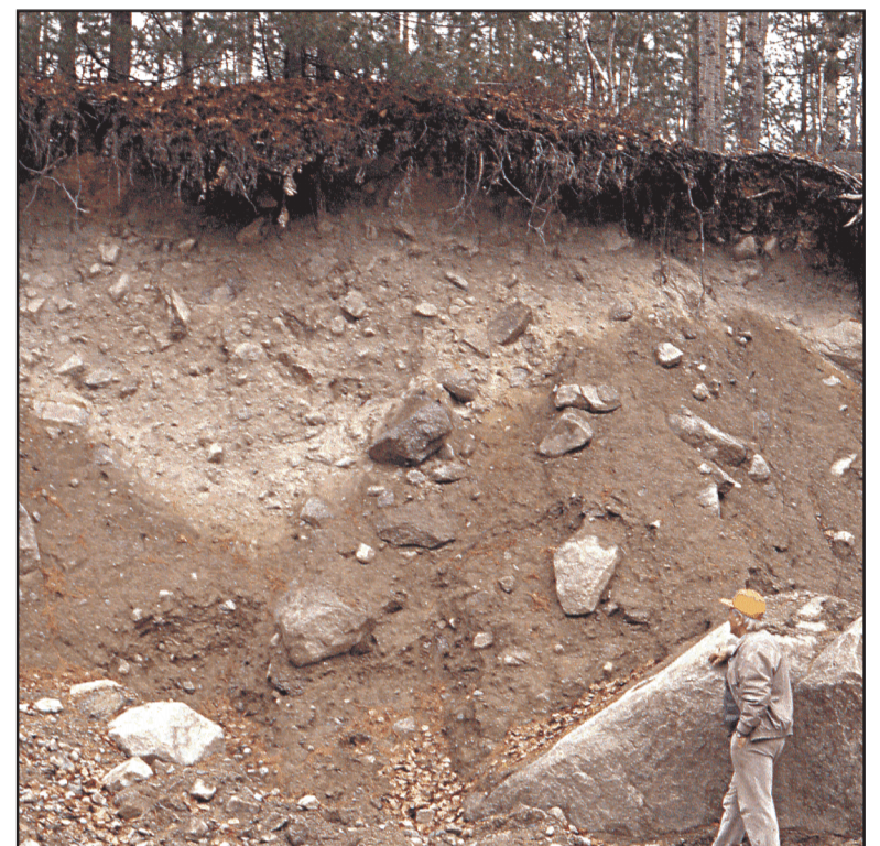
Till: ds(t) -- Borrow pit near Millinocket, exposing sandy, bouldery till. This stony till commonly occurs in areas of granitic bedrock.
