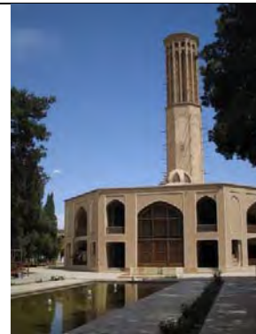
Figure 6: The windcatcher of Dowlatabad in Yazd, Iran—one of the tallest existing windcatchers
