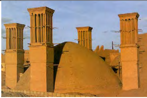
Figure 9: Reservoir with six wind tower
