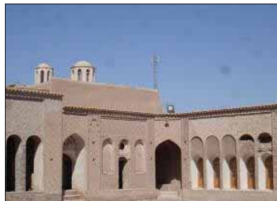
Figure 12. Southern Iwan (porch)
