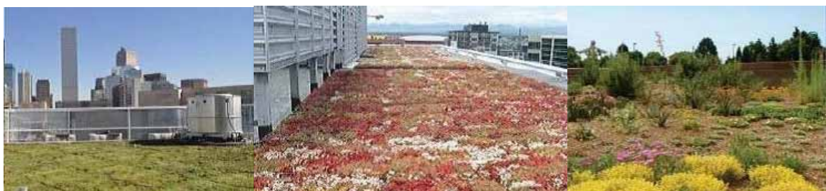
Figure 9. Types of extensive green roof, from left to right: modular trays, interlocking modular system, weakened.
