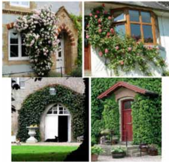
Figure 1: Left: the direct system, plants are attached directly to the wall, left indirect systems, connecting green facade by support structures
