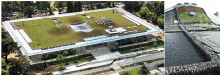
Figure 10. Green Roof in the California Academy of Sciences and its infrastructure
