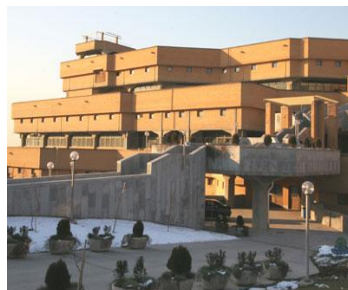
Figure 4. National Library building
