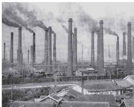
The central boiler zone
