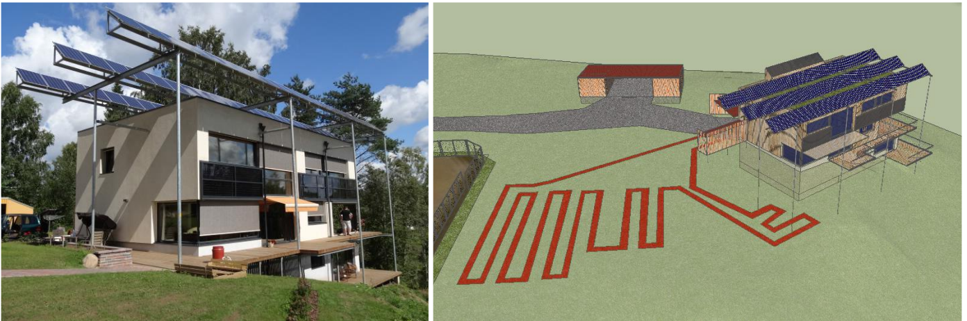
Fig. 1. View from the SW direction (left) and position of the pre-heating system ground loop (right).
