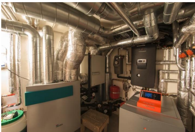
Fig. 3. Ventilation unit (left) and ground source brine heat exchanger (right).
