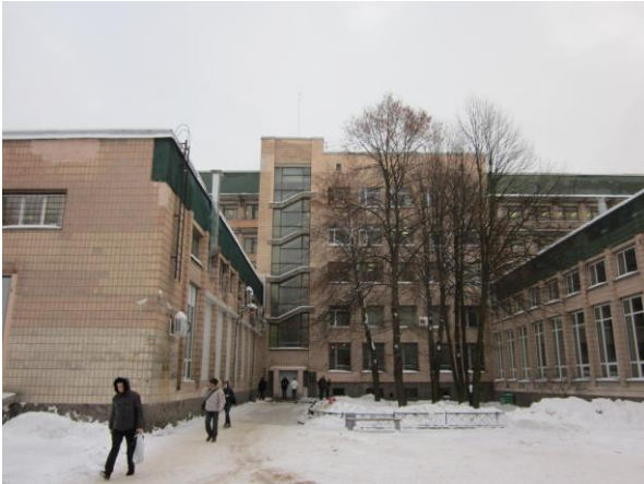
Fig. 3. "Hydrotechnical building-2" at the campus of SPbSTU.
