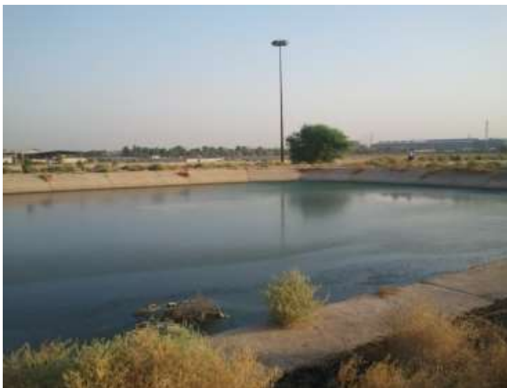
Figure 1. A view of stabilization ponds of Ahvaz's slaughterhouse
