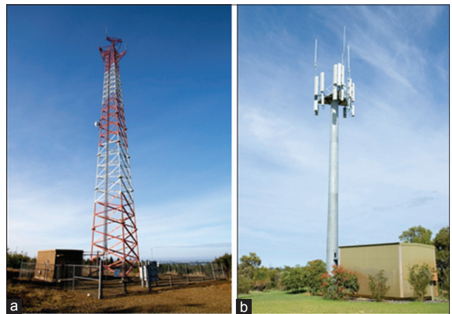
Figure 1. Photo of (a) latticework structure tower, and (b) monopole structure tower. Photos are taken from: http://www.fructivore.com/2010/10/look-for-the-right-short-candidates-like-crown-castle/ , http://commons.wikimedia.org/wiki/File:Telstra_Mobile_Phone_Tower.jpg .
