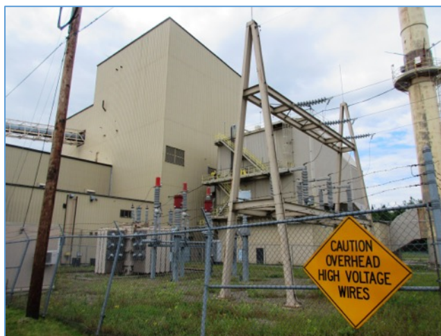
Former Covanta Biomass Energy Plant
