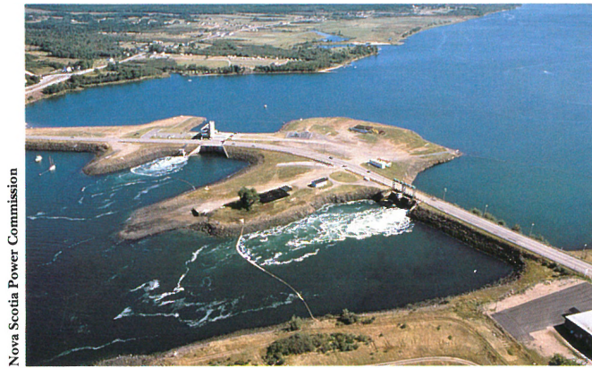
The tidal power plant that currently operates on the Annapolis River in Nova Scotia has affected local current patterns, caused upstream riverbank erosion, killed fish passing through the turbines, altered the natural deposition of sediments, and influenced the soft shell clam fishery in the Annapolis Basin.
