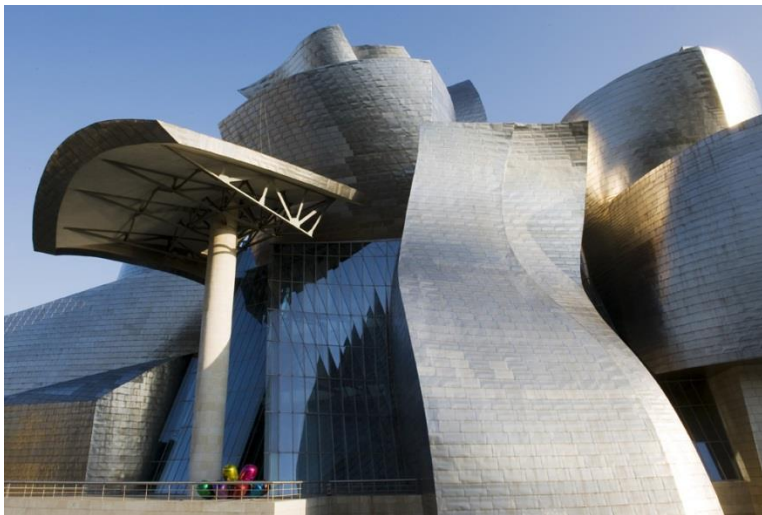
Figure 16: Exterior detail of the Guggenheim Museum by Frank Gehry
