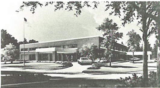
The Architectural Conception of H.A.D. No. 4 Hospital Under Construction in 1976.
