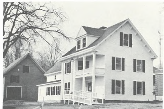
Court House Annex This annex will house District Court 13, the Judge's Chamber, Clerk of Courts, the Law Library, District Attorney Office, and other accommodations.
