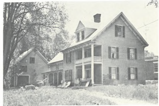
Joseph B. Peaks House Before Renovation for Maine District Court.
