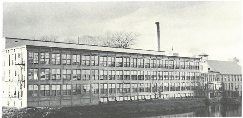
Former Mayo's Mill, Now Moosehead Furniture Manufacturing Company.
