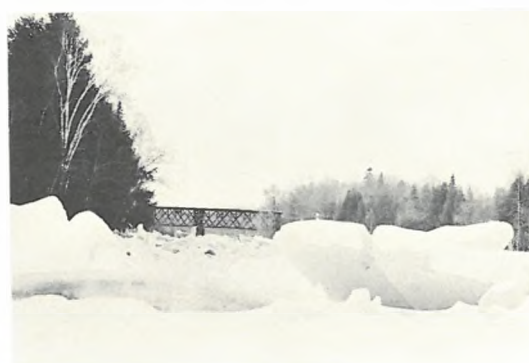
Railroad tressle over Piscataquis River and big ice jam, 1970.
