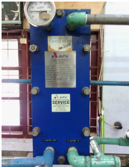
Gambar 4. Rangkaian Alat Penukar Panas Plate and Frame Tipe TRIGMS 10
