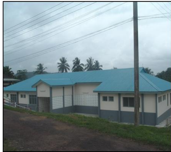
Plate 2: Maternity Block at Tarkwa
