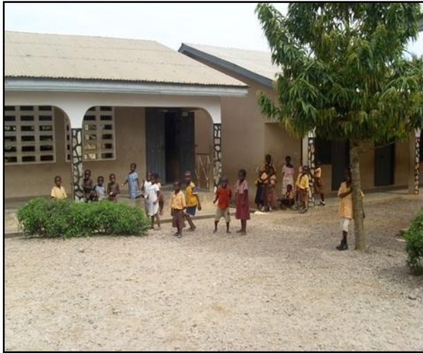
Plate 1: A New Classroom Block at New Atuabo
