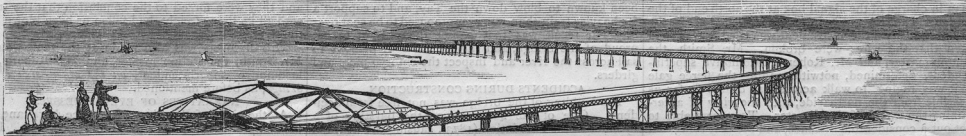
VIEW OF THE TAY BRIDGE BEFORE THE ACCIDENT.
