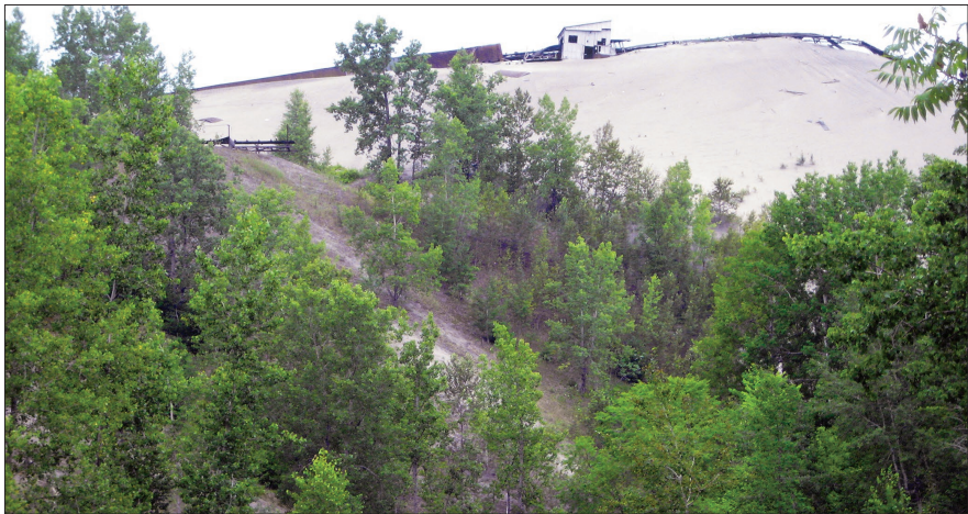
Figure 3: Tailings at Mineville, Essex County.
