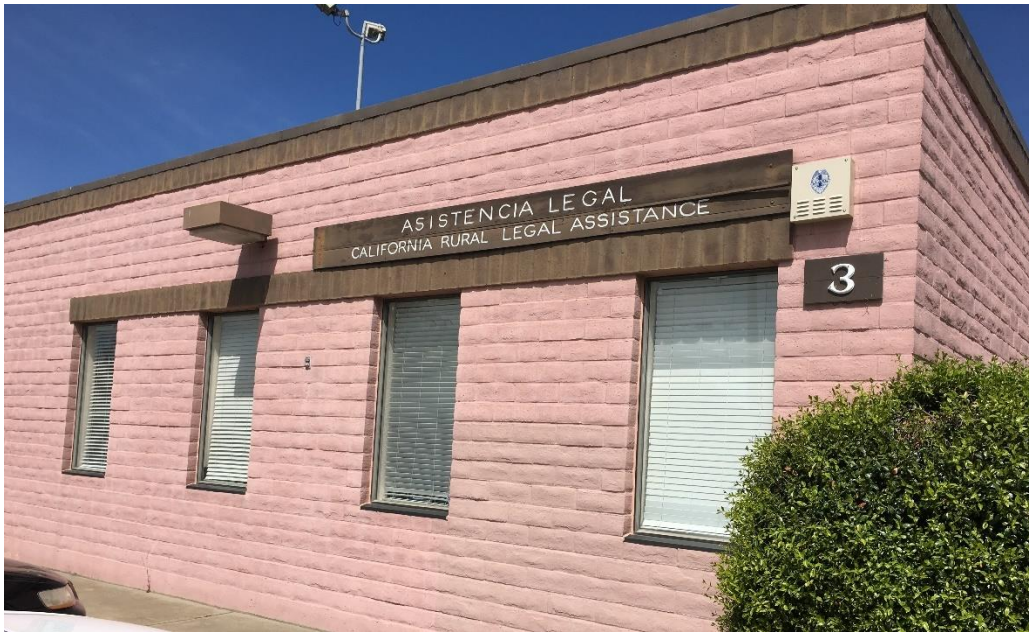
Front view of CRLA building located in Salinas, California. ©Jonathan Chavez
