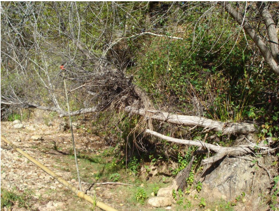
Figure 16. Irrigation pipeline installed by the MPWMD as part of the RHP in the Quail to Via Mallorca survey area. The LWD on the right was outside the active channel, but recorded due to its high recruitment potential during a high flow event.
