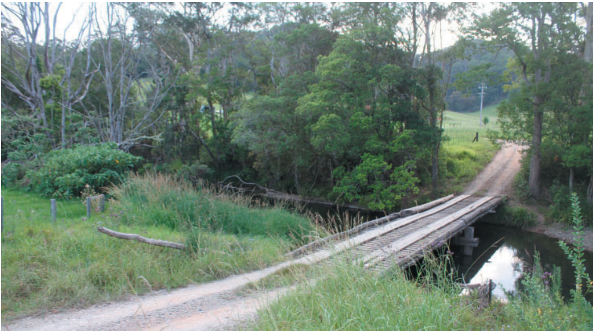
Fig. 3. Bridge across the Orara River, on original site of Hoschke's farm on the other side of the river. Doug Hoschke, grandson of the original farm owner, took Dan Lunney to this site, as he knew both the old photo and the site of what was his grandfather's farm. The farm is no longer in the family. Note the regrowth along the river bank, the cleared land in the background, and the forest on the hills. Photo by Dan Lunney (3 January 2014).
