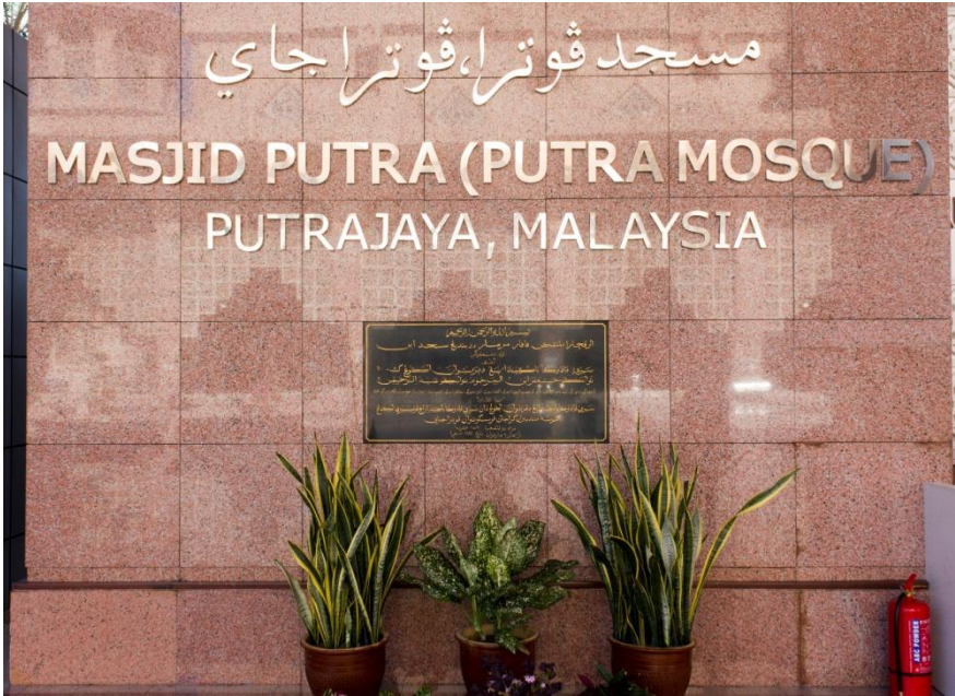
Figure 5: Masjid Putra (1999), Putrajaya, Malaysia, foundation panel (Photo: Bernard O’Kane)
