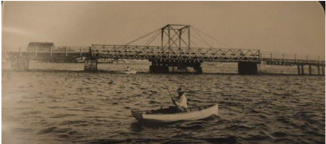
Image: Undated photograph of the Padanaram bridge and causeway. Courtesy of the Dartmouth Historical Commission.
