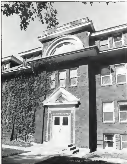
Swallow-Robin hall (left) still stands today, although it was closed as a residence facility following the 1985-86 school year. It is one of only two buildings built before 1950 which remain structurally the same as when originally built, the other being Sickler Hall, erected in 1902-03, which faces Swallow-Robin across Reade Avenue.
