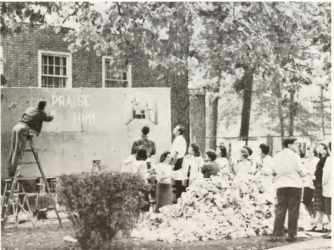
Erecting a Home Coming Display
