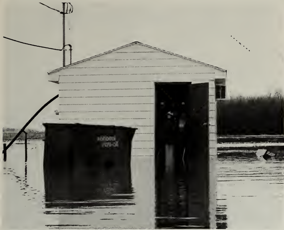
A foot and a half of water filled the transmitter building during the flood in March, but none of the equipment was damaged.
