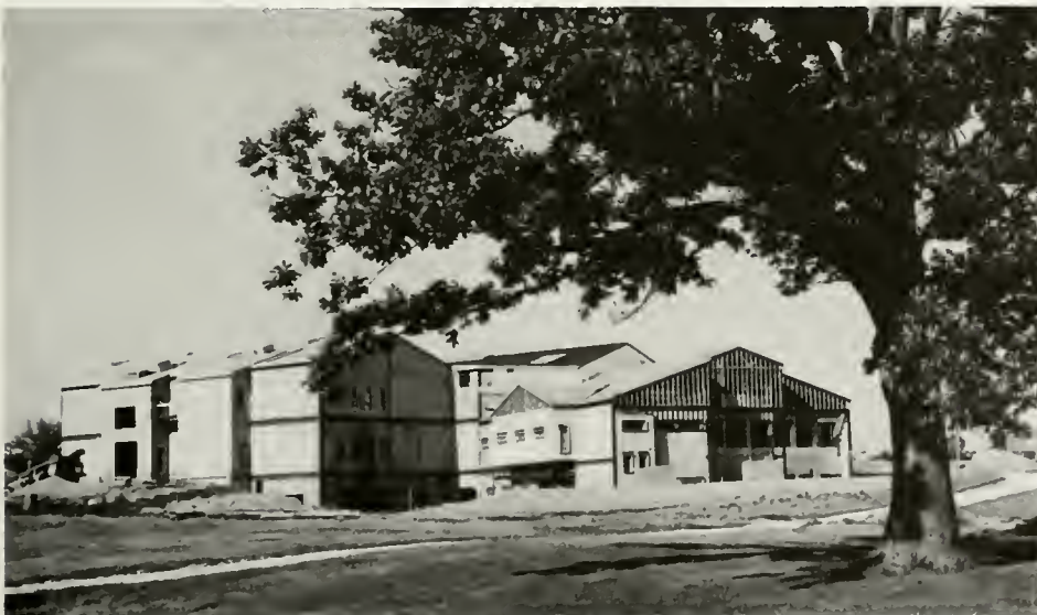
Zondervan Library Nearing Completion
