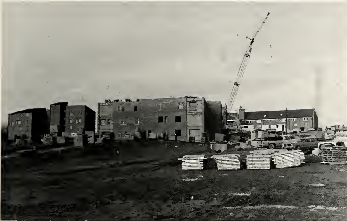
Taylor's community expands through the construction of a new dorm.
