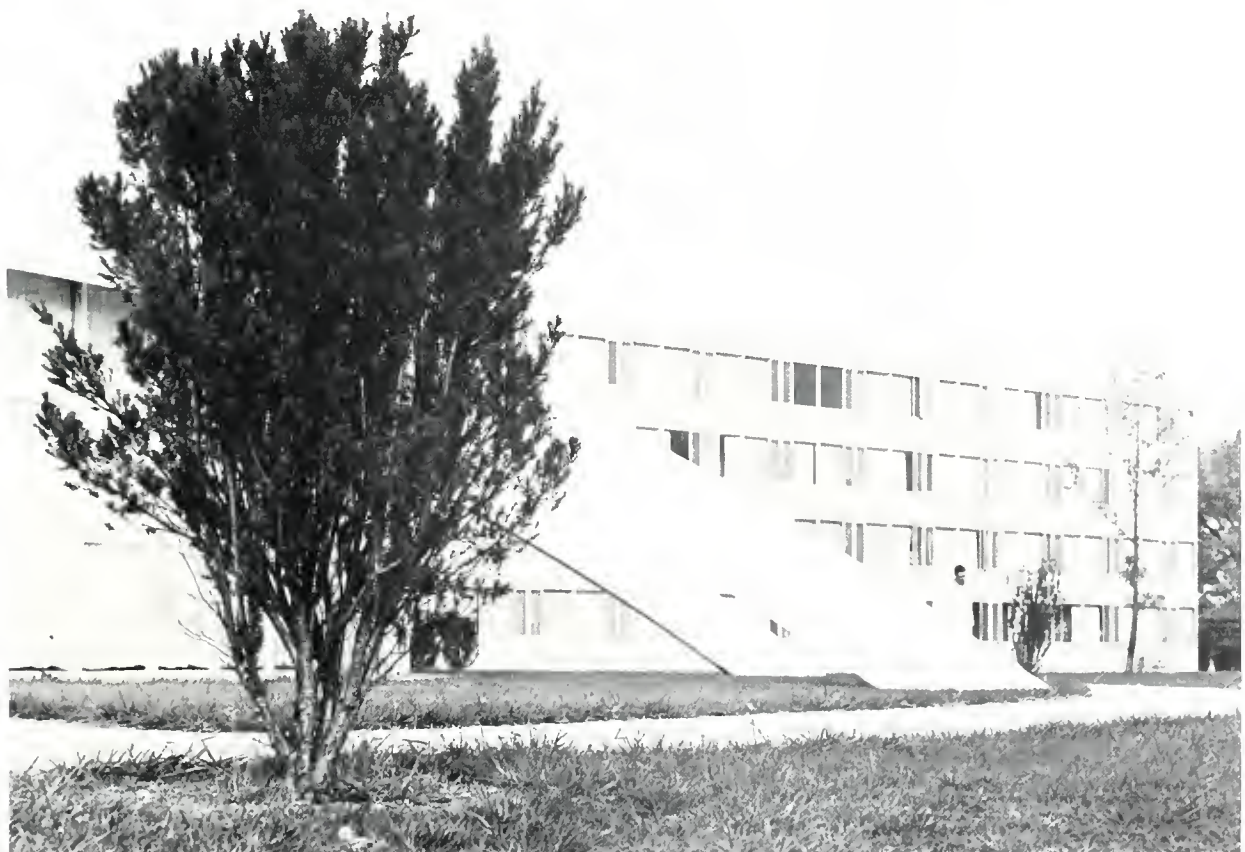
MORRIS DORMITORY is seen around the corner and under the beams.
