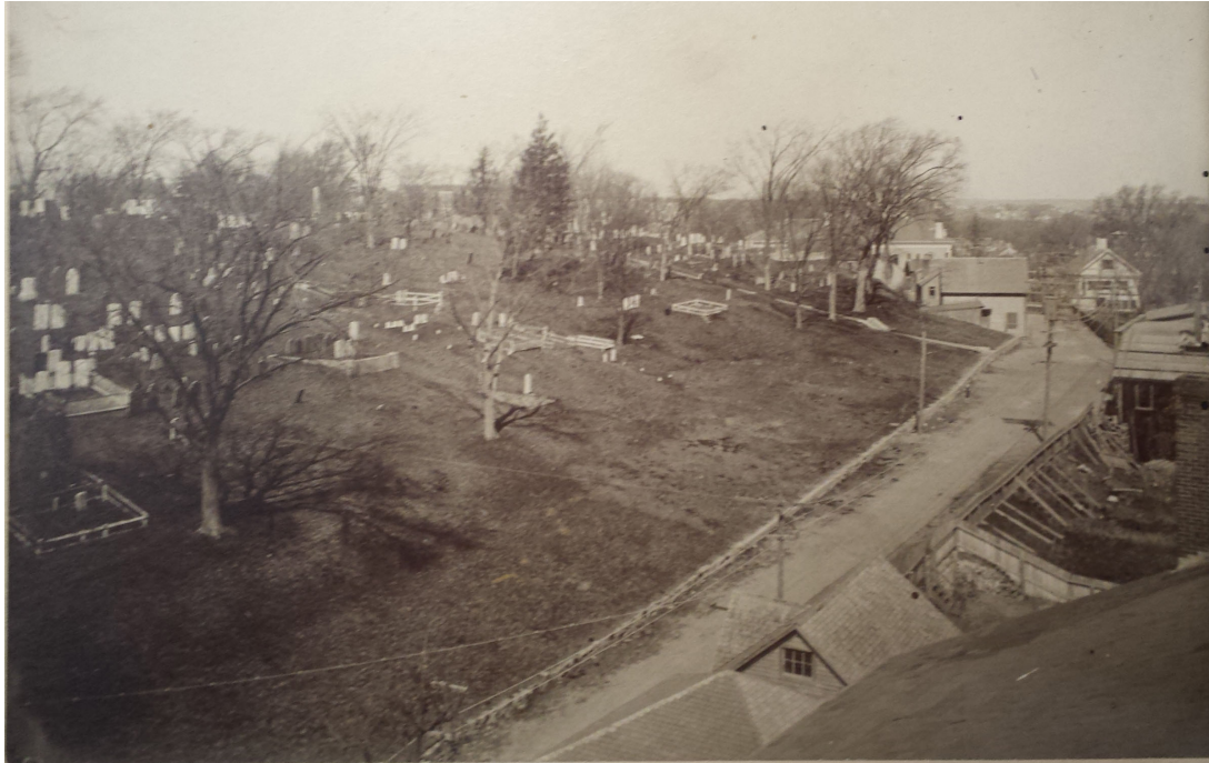
Figure 6. Photograph taken after the demolition of the stable buildings and school on School Street, looking north, before the area had been fully filled and graded.
