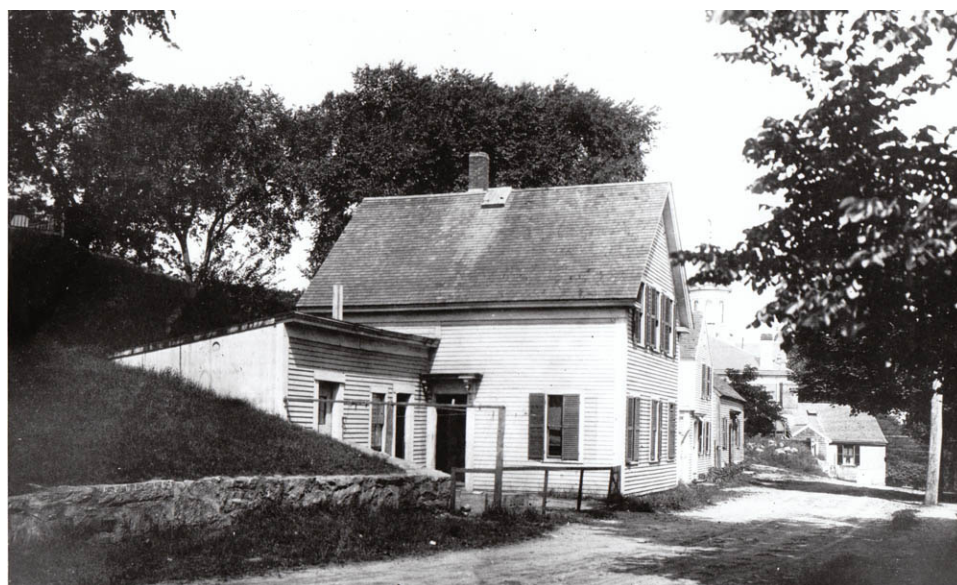
Figure 15. Residential buildings on School St., showing how the buildings were cut into the hillside (Baker and Keith 2013: 8).
