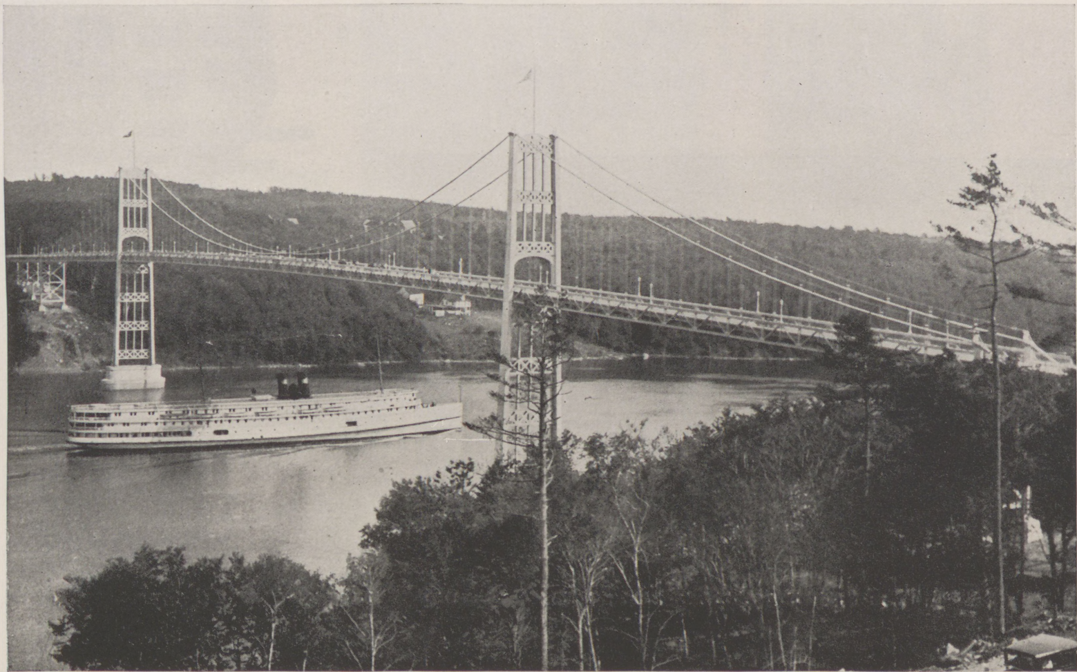
The Waldo-Hancock suspension bridge on coastal route No. 1 over the majestic Penobscot River, connecting the towns of Bucksport and Prospect, 19 miles below Bangor
