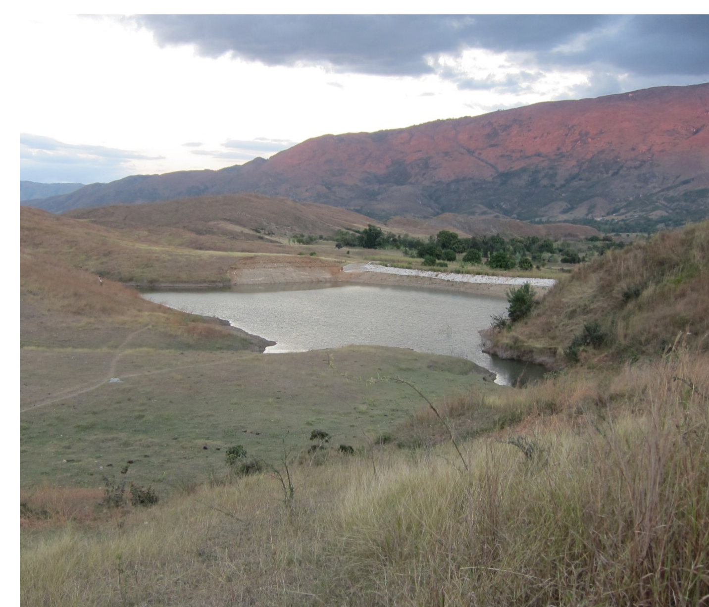
Reservoir and fish farm
