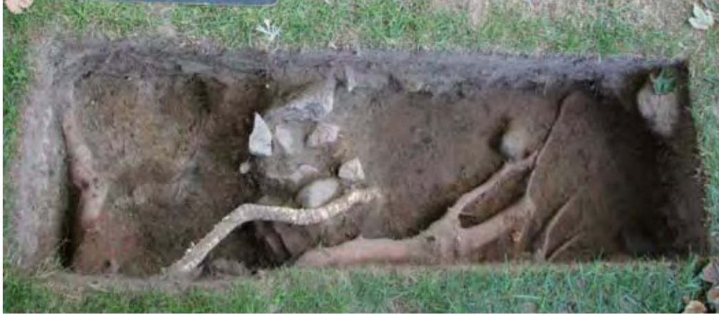
Figure 4.4: West sill support of the western addition in JTP 1, facing north.
