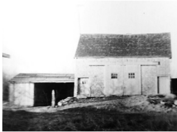
Figure 3.18: 19th century barn. Only the foundation remains. (Courtesy Muriel Bibeau.)
