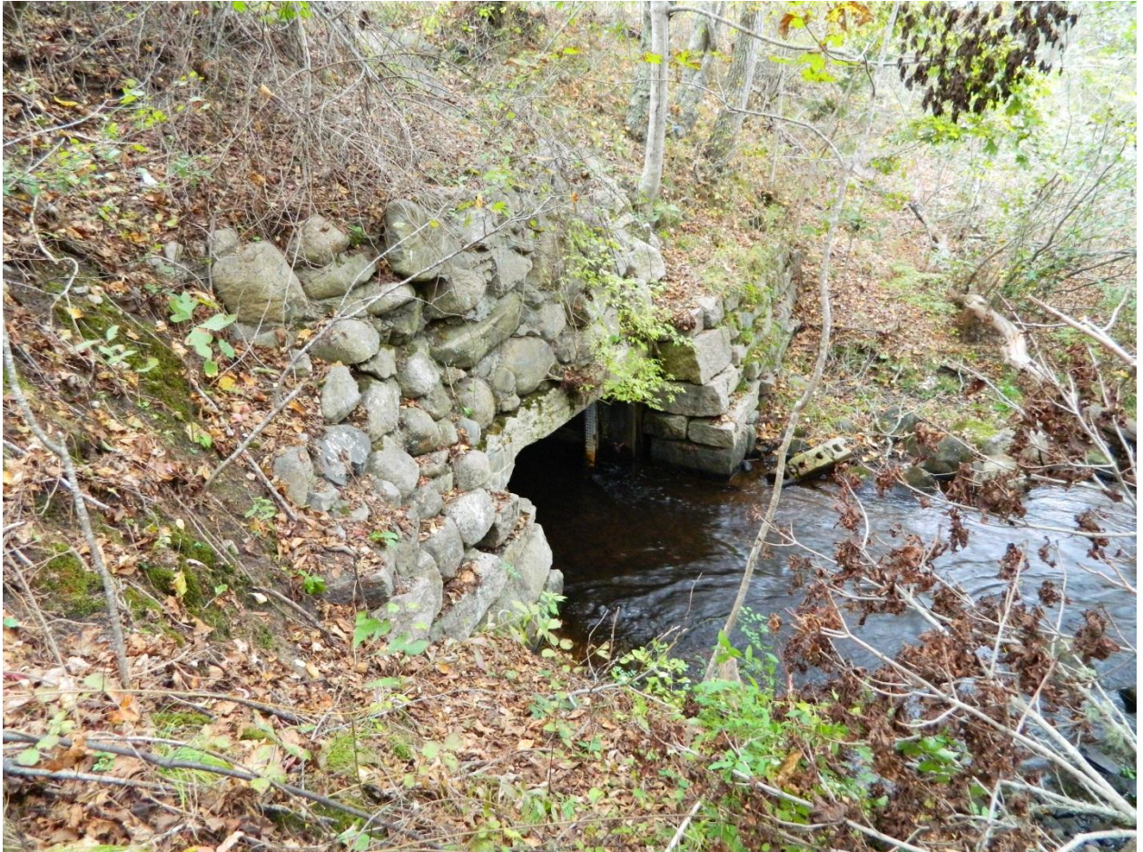
Figure 5. Remnant wheel head on the south side of the Moonakis dam. Picture taken by Leo Patrick Ledwell, Jr.
