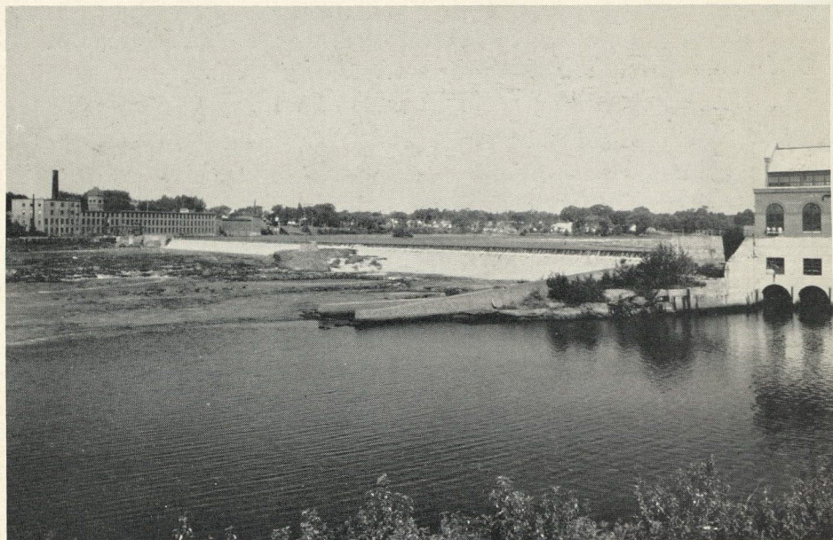
OLDTOWN DAM ON THE PENOBSCOT, OLDTOWN
