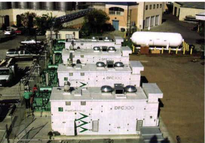
■ The installation of four DFC300 high temperature, high-efficiency carbonate fuel cells provide the brewery virtually all of its baseload electrical power. >> Photo courtesy of Sierra Nevada.
