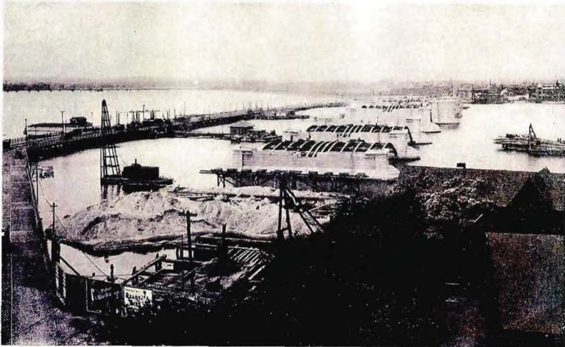
Fig. 9. Steel arches and piers in place, 1904
