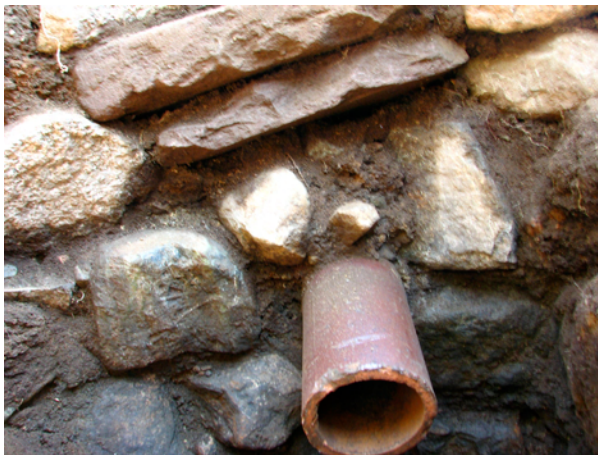
IV.53. Drain pipe entering the north wall of Feature 1.
