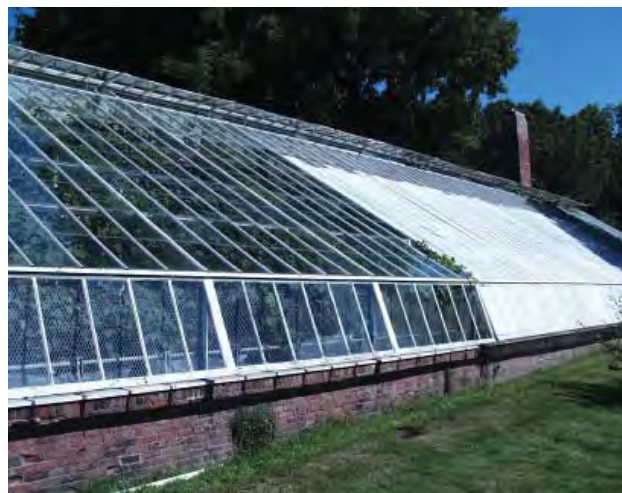
Figure 3.5. A) Profile of a greenhouse with a substantial back wall and short front knee wall from Diderot's Encyclopedie ; B) Detail of greenhouse at the Vale using this construction method.
