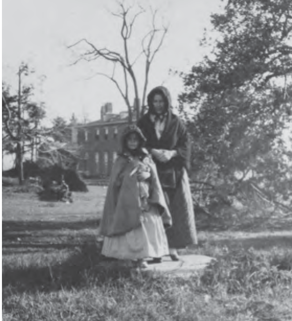
Figure 2.22. Photo of ca. 1927 depicting the two stones that cover the well.
