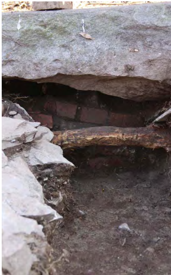
Figure 2.25. Brick wall of well (facing east).
