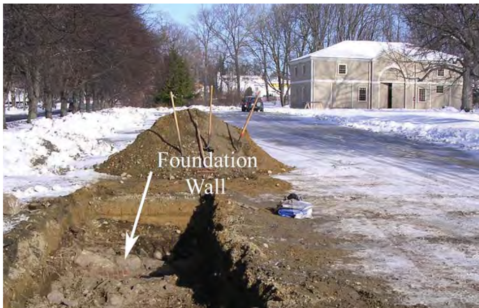
Figure 2.12. Excavation trench and north wall location in 2004 (facing north).
