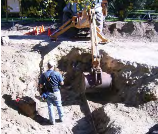
Figure 2.15. Backhoe removing fill from carriage house cellar, facing east.
