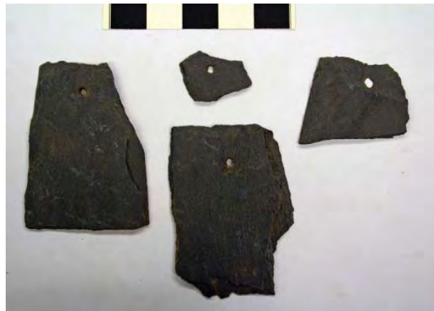
Figure 5.3. Roofing slate with nail holes. Photograph by Heidi Krofft.
