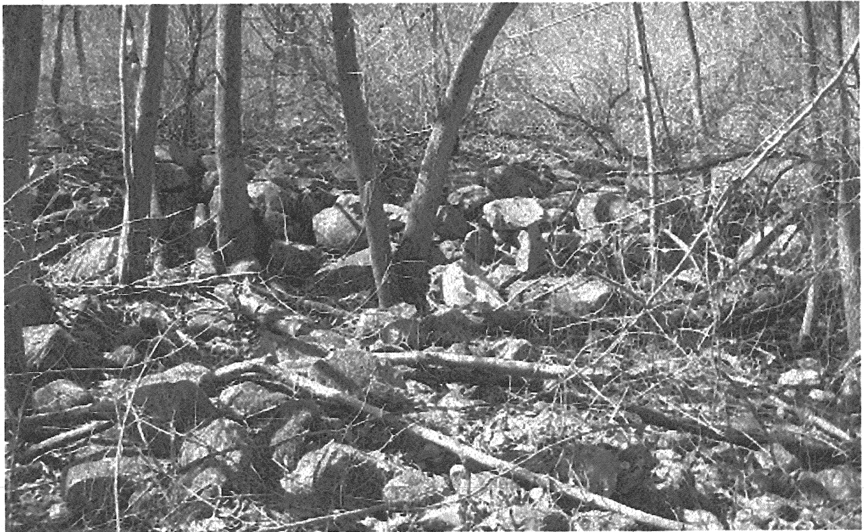
Photo 14: Cobbled Surface 1, Looking West Showing Eastern Retaining Wall
