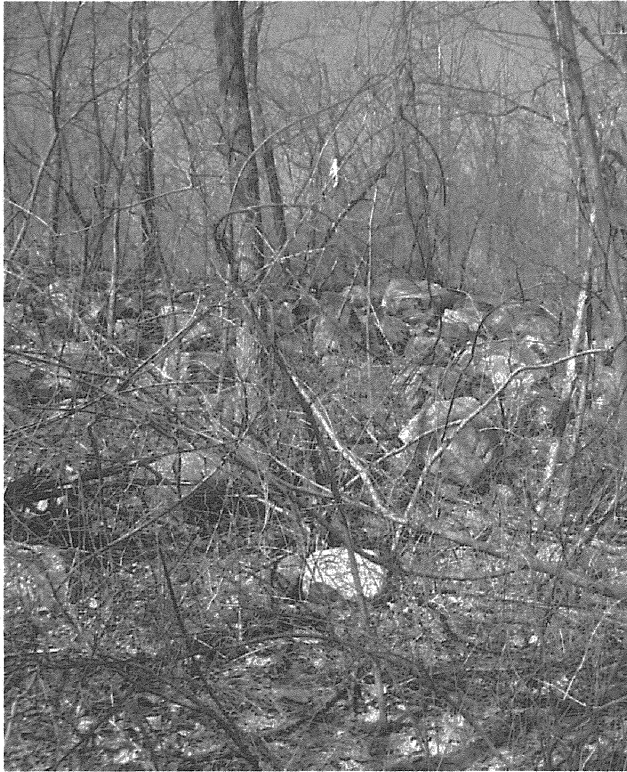
Photo 20: Retaining Wall, Looking West
