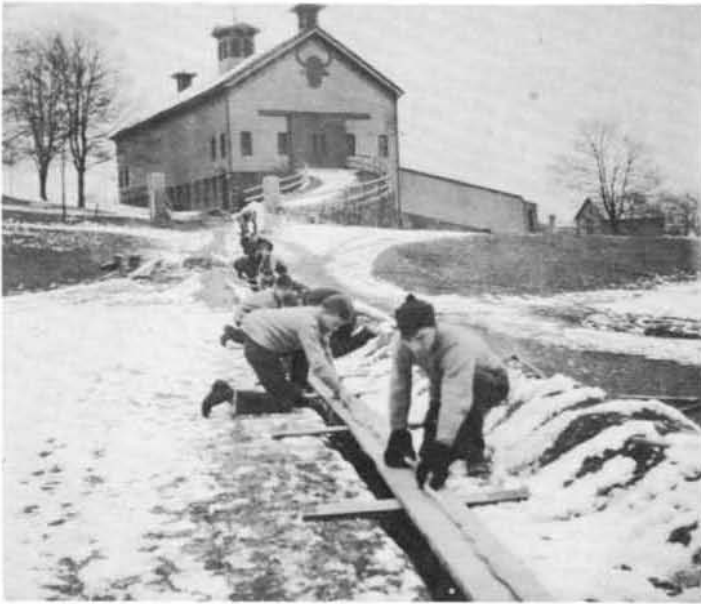
Students laying electrical cable from barn to pier, 1914
