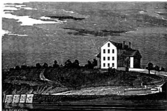
Main building and stone pier, c.1840
