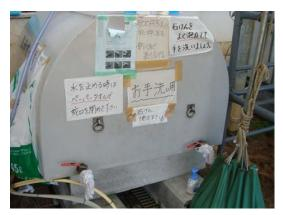
Tank from small water supply vehicle was settled on the ground and refilled with water every morning
