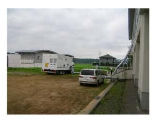
Cool air is blowing into gymnasium from air conditioning vehicle
