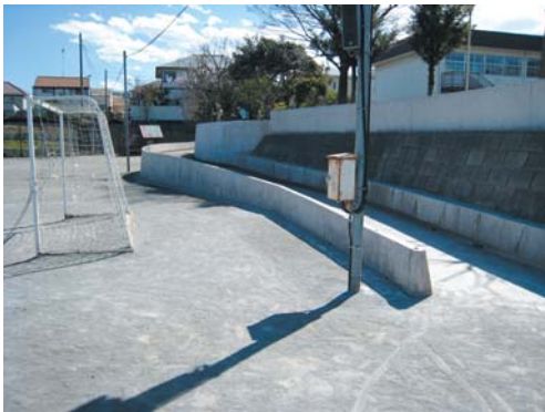
Slope to outside ground
