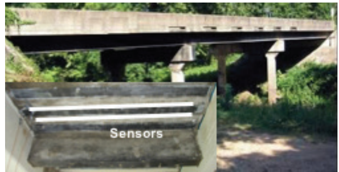
Fig. 1: The Dallas County Bridge with two instrumented sensors
