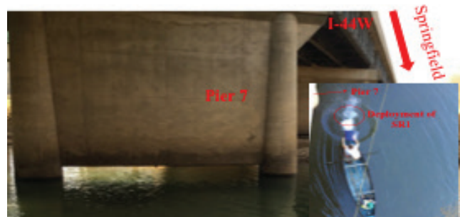
Fig. 2 The Roubidoux Creek Bridge with smart rock (SR1) installation
