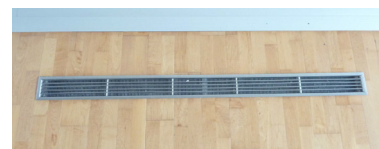
Blowing slits on the floor surface
