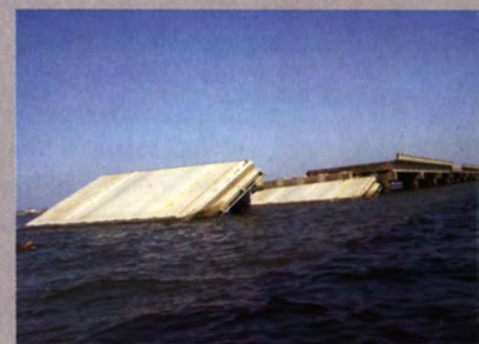
Twin span bridge of Interstate 10.
