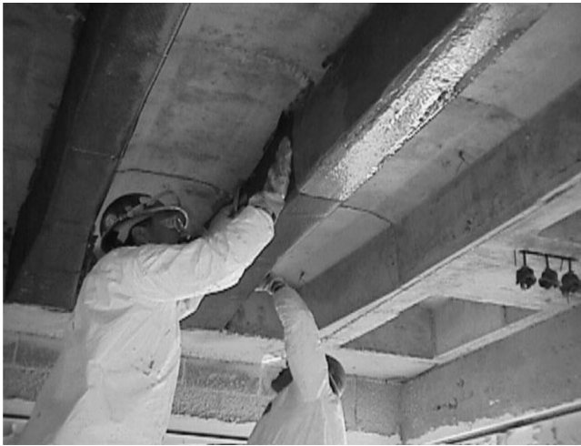
FIGURE 1 Application of FRP sheet on one-way joist.
